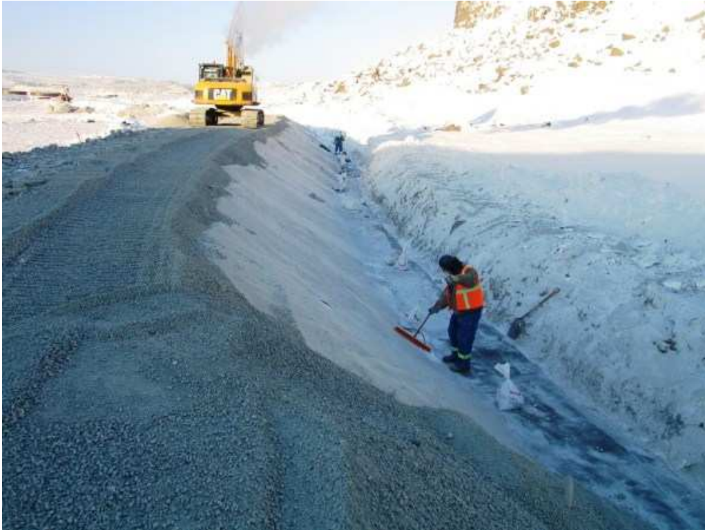
Photo 6: Labourers removing snow in key trench.
