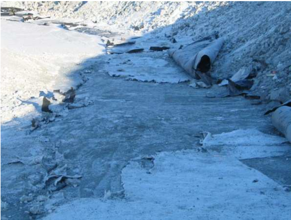
Photo 7: Cleaning at south end of berm. GCL was ripped and removed at this location
