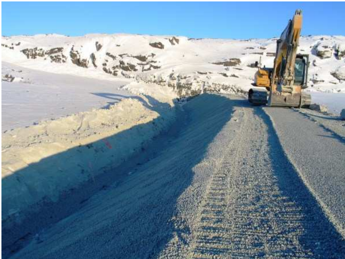
Photo 2: Progress on the north diversion berm. Bentonite was placed over HPDE. \frac{3}{4} " crush placed on top of berm and slopes. Section from 0+585 to the end.
