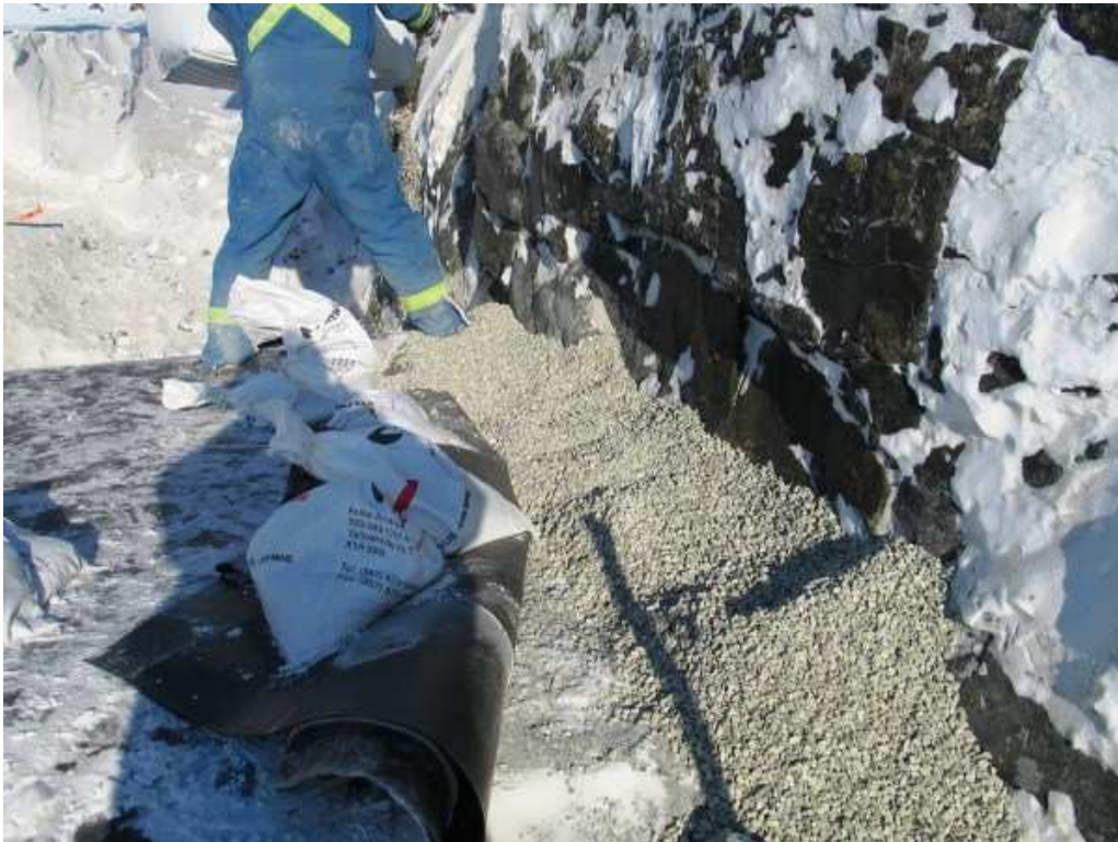
Photo 5: Bentonite seal placed at end of berm (tie in to rock face)
