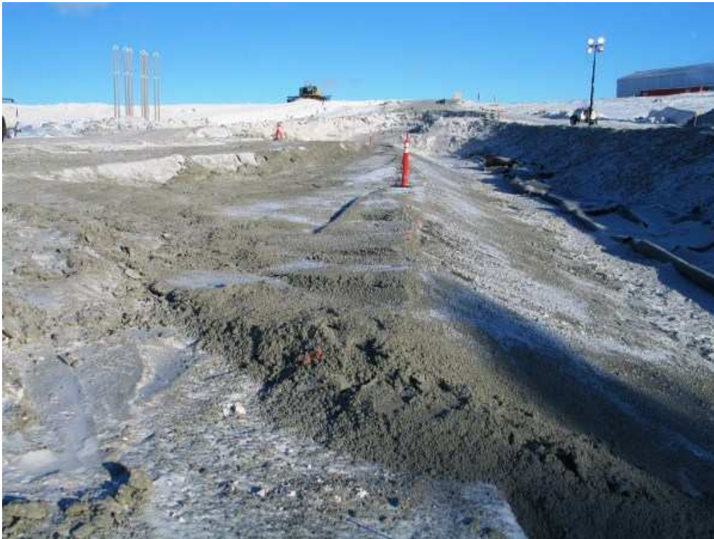
Photo 8: Slope at the north end, Sta 130. FCM placed March 1 st nightshift.
